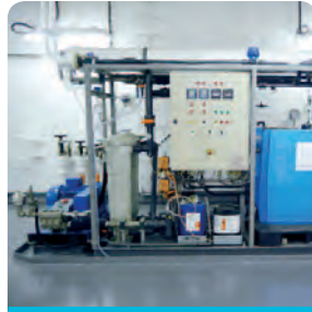
Hatenboer-Water RO system on board Transocean drillship
